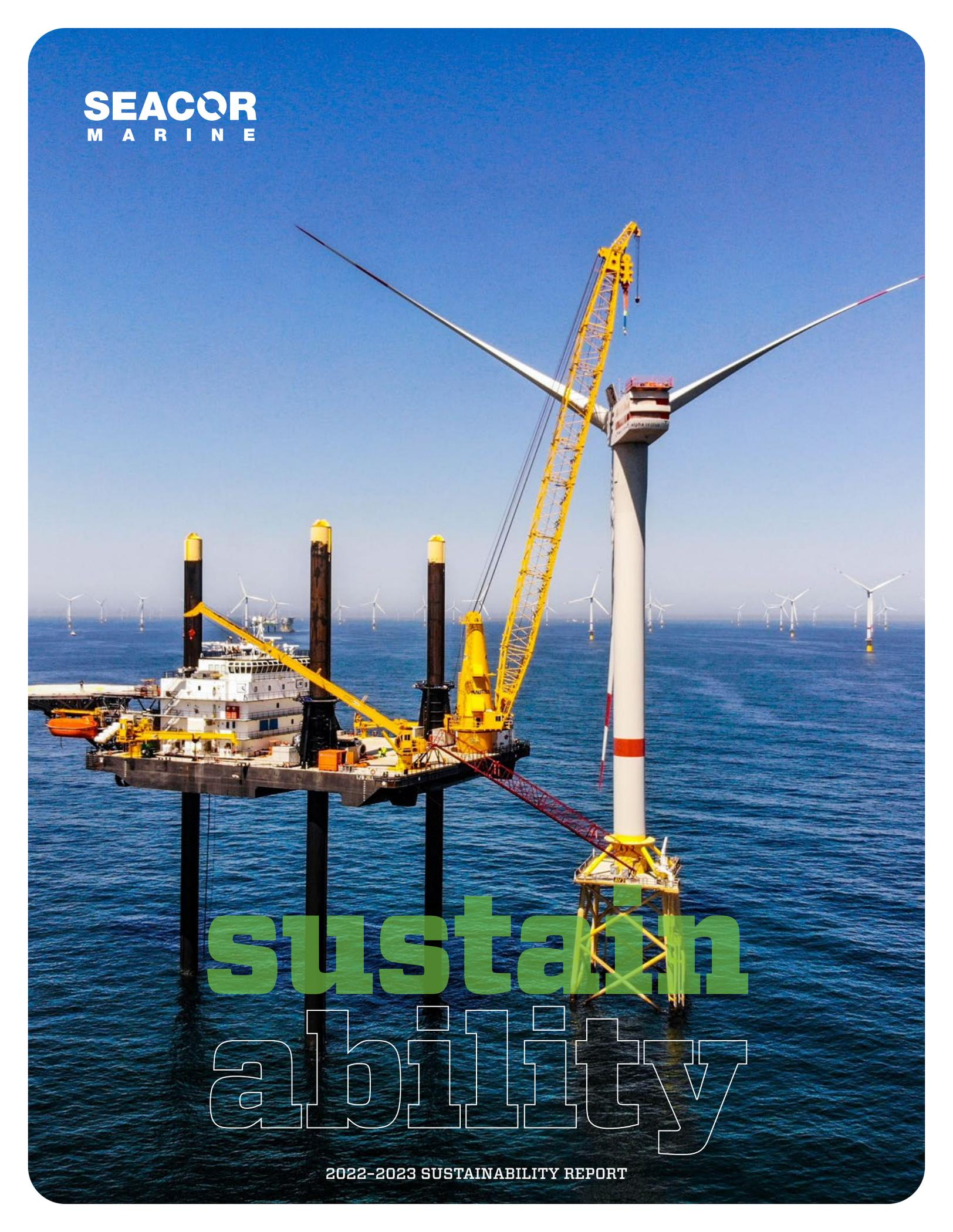
A large-scale photograph of an offshore wind turbine installation. A yellow crane is mounted on a platform, lifting a white turbine tower section. The platform is supported by several black piles in the blue ocean. In the background, many other wind turbines are visible on the horizon under a clear blue sky.
